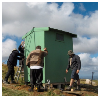
Hut back on its new foundations
