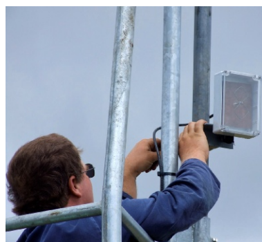
Preparing the enclosed dipole antenna for our 12cm beacon
