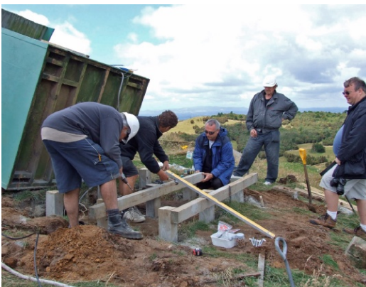
New foundations being prepared for hut
