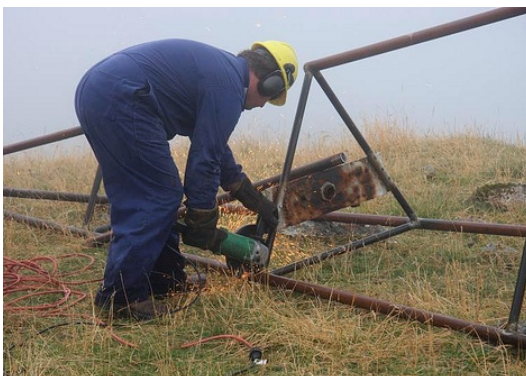
Cutting up the old tower for scrap
