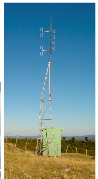
Installation all complete
