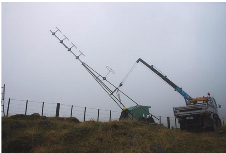
The old tower being lowered in the mist and drizzle
